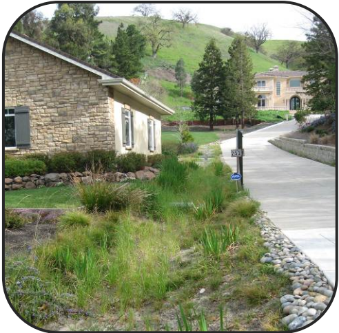
Large Residential Rain Garden
